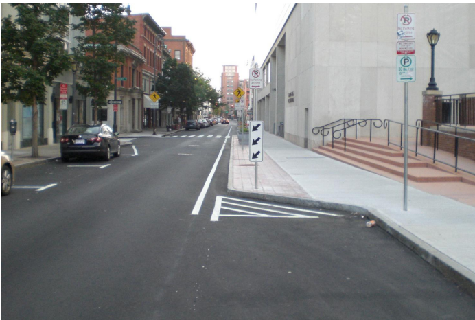
Bump-out along Orange Street. Source: www.pedbikeimages.org / Tom Harned
